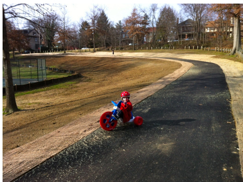
New benches and a new walkway in Tyler Park. Read about it in the "View from the Bridge" on page 2.
